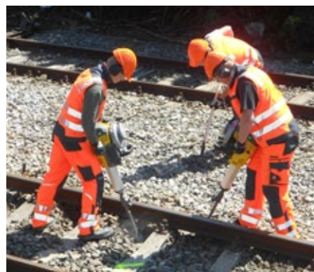
The BH40 and BH55rw gasoline breakers are specially optimized for maintenance work in railway track construction.
